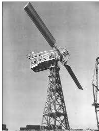
Figura 2 - Turbina Smith-Putnam 1941 USA
