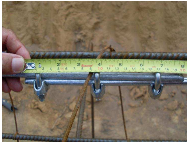
Figura 6 - Conexão de 20cm entre as RE-BARS.
