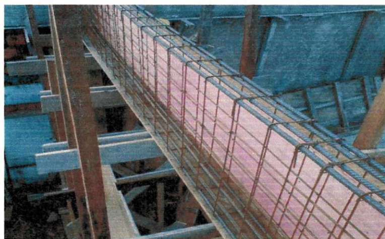
Figura 4.13 – viga com painel lateral
