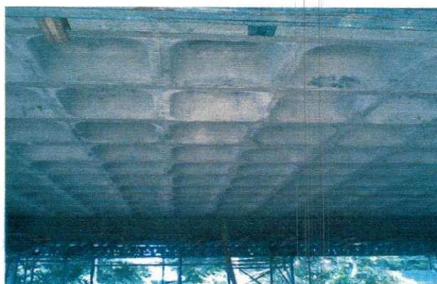
Figura 4.4.6 – Laje nervurada pronta
