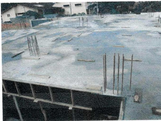
*Figura 16, Figura 17 e Figura 18 – Laje concretada.*
