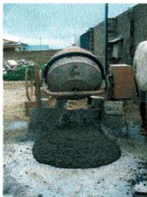
Figura14 – Concreto fabricado in loco
