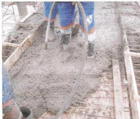
FOTO 58: CONCRETAGEM DA LAJE
