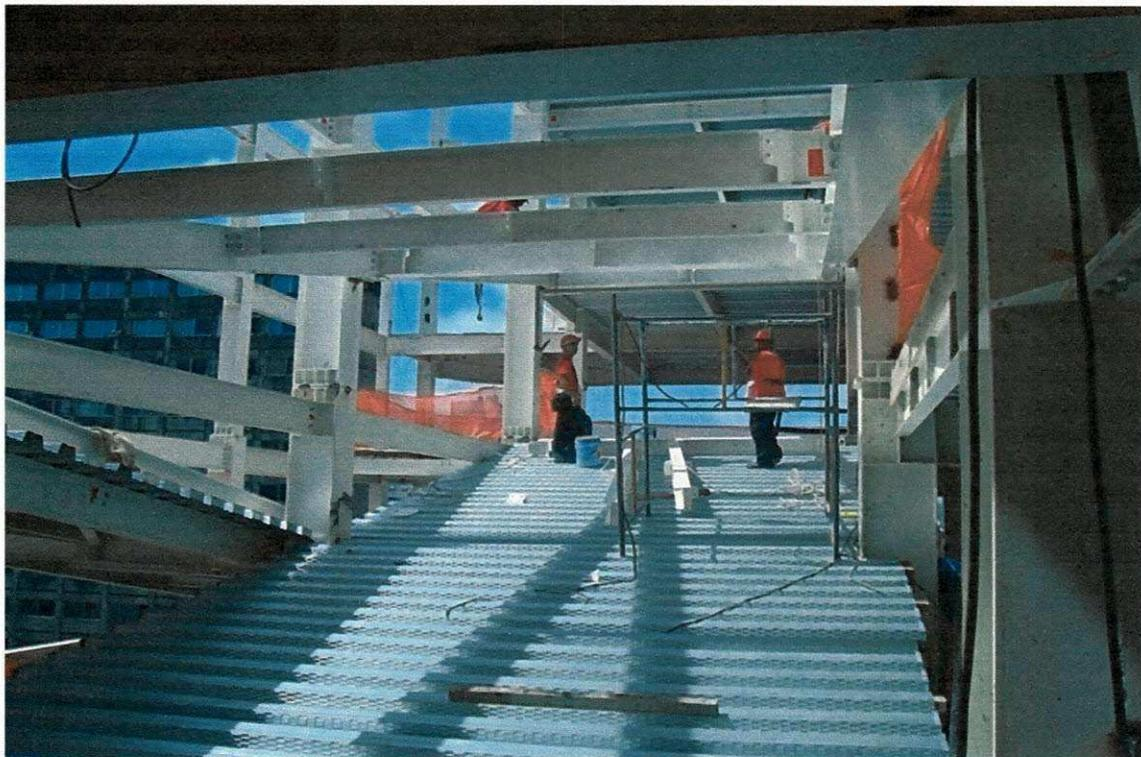
**Figura 67 - Rampas com lajes steel decks.**
