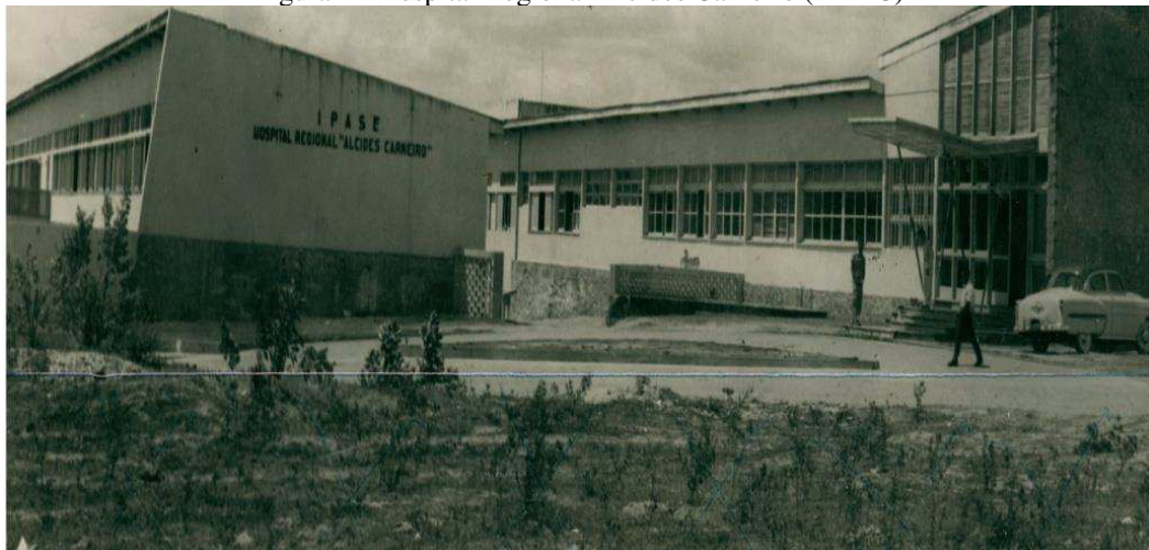
Figura 4 - Hospital Regional Alcides Carneiro (HRAC)
