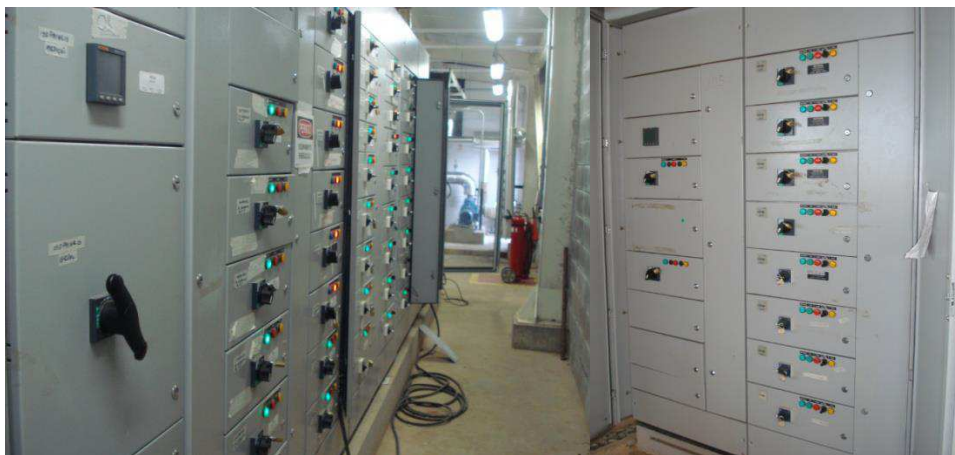
Figura 4.13 – Painel CCM FTS e Painel UOS
