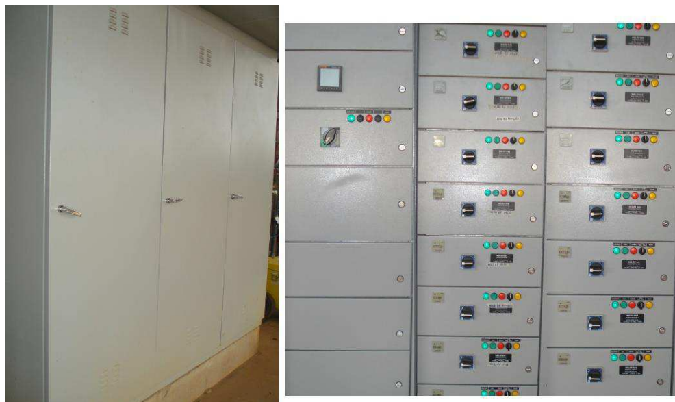
Figura 4.11 – Painel CCM DASR 5.
