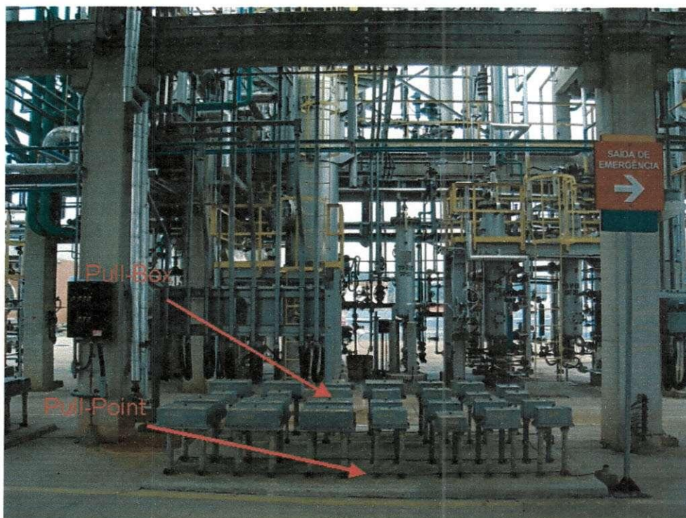
Figura 16. Pull-Point e Pull-Boxes
