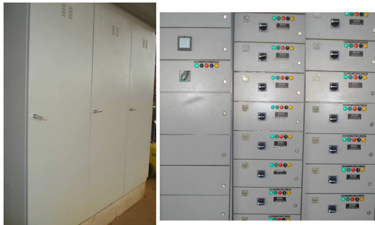
Figura 14 – Vista frontal do Painel CCM DASR 5.
