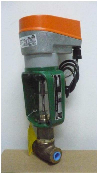
Figura 5.12: Baumann NV electric actuator.
