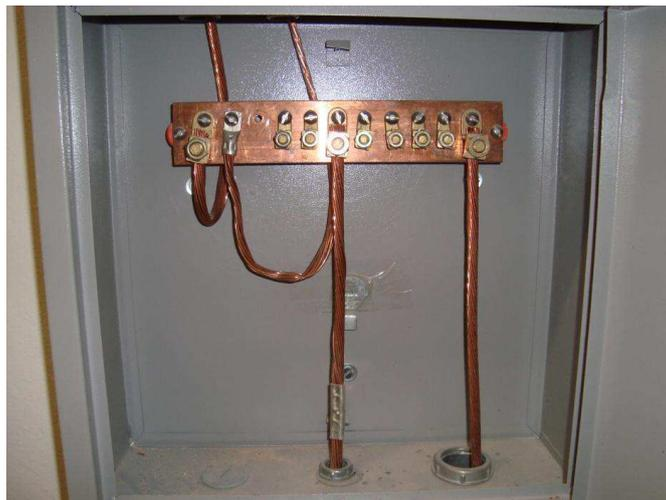
Figura 14 – BEP Instalado
