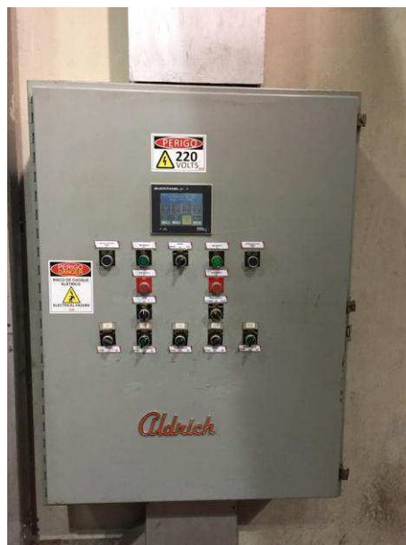
Figura 21 - Painel com as botoeiras antigas.
