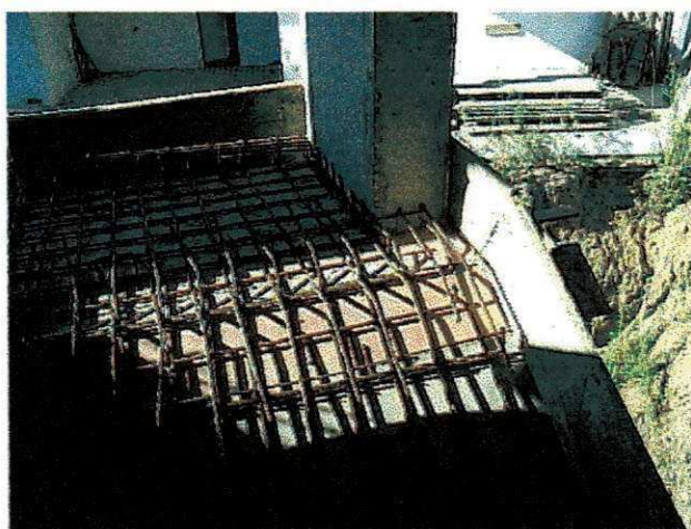
Figura 25: Armadura principal
