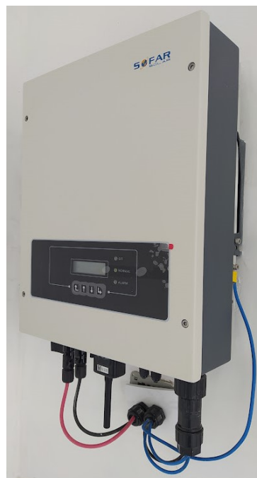
Figura 17 – Inversor Solar Grid-Tied Sofar 4KTLM-G2
