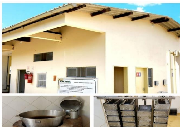
Figure 1 – Standardized architectural structure and stainless equipment of family agro industries, producers of artisanal coalho cheeses, in the state of Rio Grande do Norte, Brazil.
